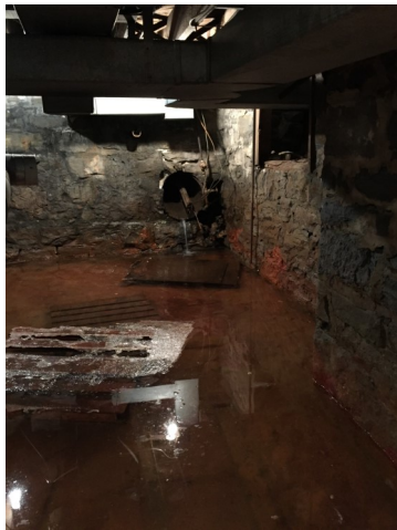
Before photo of the basement
