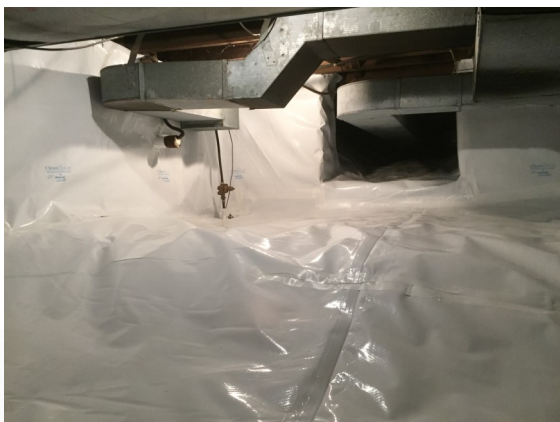
Completed basement project
