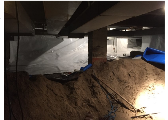
In progress photo
