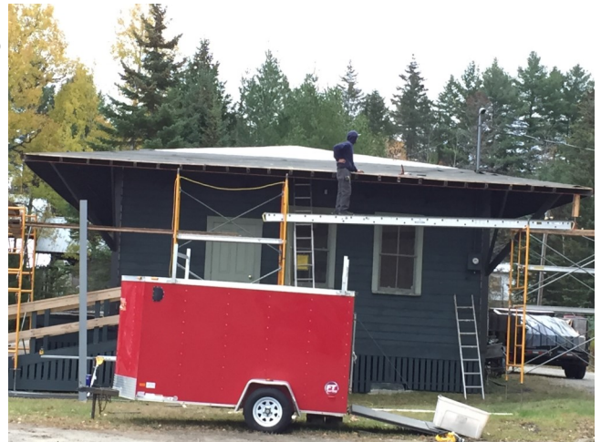
In progress photo of the Freight House being repaired
